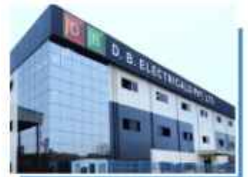
D. B. Electricals
